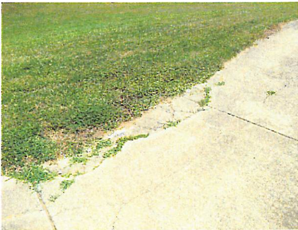
Organic growth in concrete cracks
