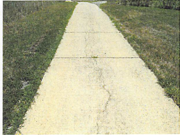
Concrete center line cracks
