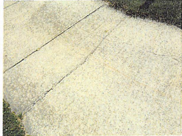
Sidewalk crack
