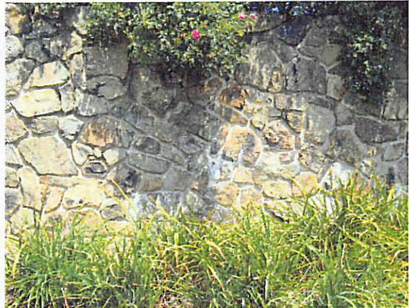
Efflorescence evident
