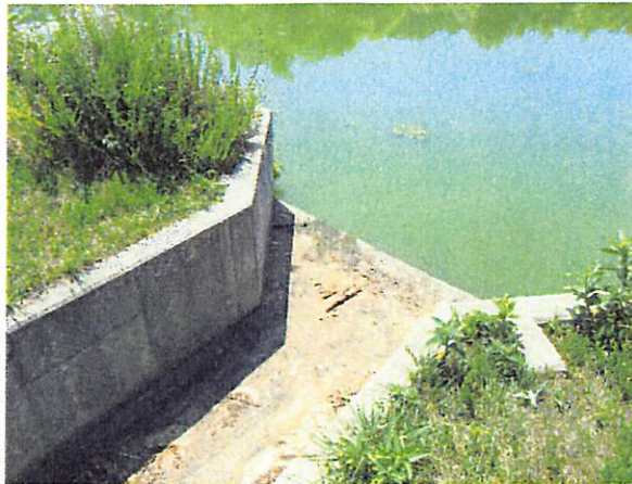
Concrete outlet structure
