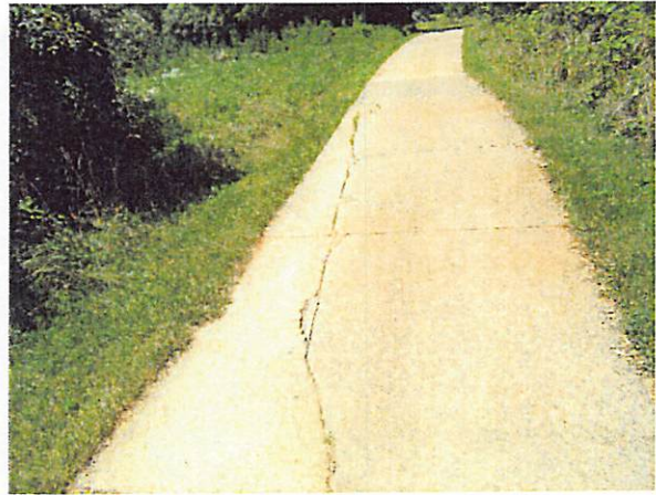
Concrete crack
