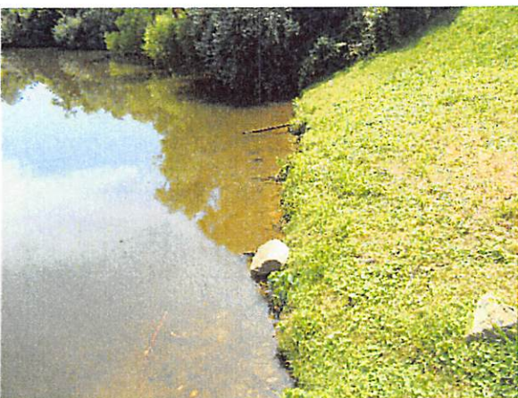
Erosion evident at Pond 2
