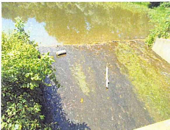
Sediment accumulation evident at Pond 6
