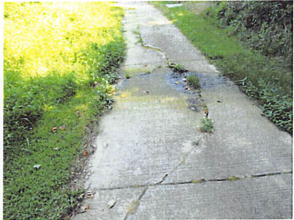
Concrete cracks and organic growth
