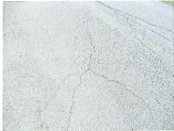
Cracks at Count Turf
