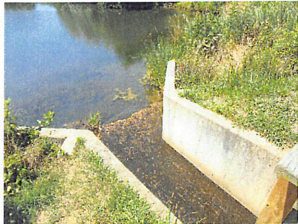
Sediment accumulation at Pond 4
