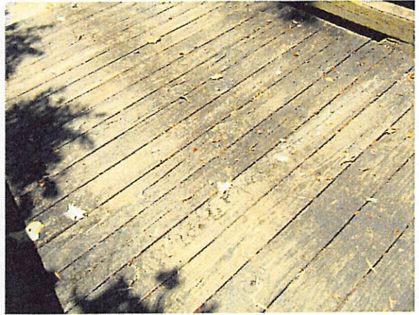
Wood deterioration
