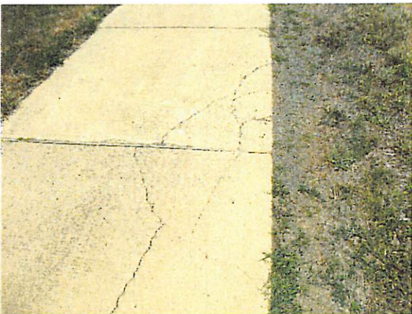
Concrete cracks
